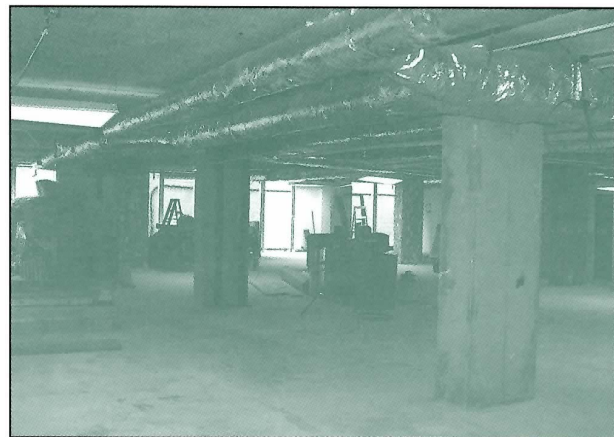
Construction begins on the 2nd Floor of the Wisconsin Veterans Museum
